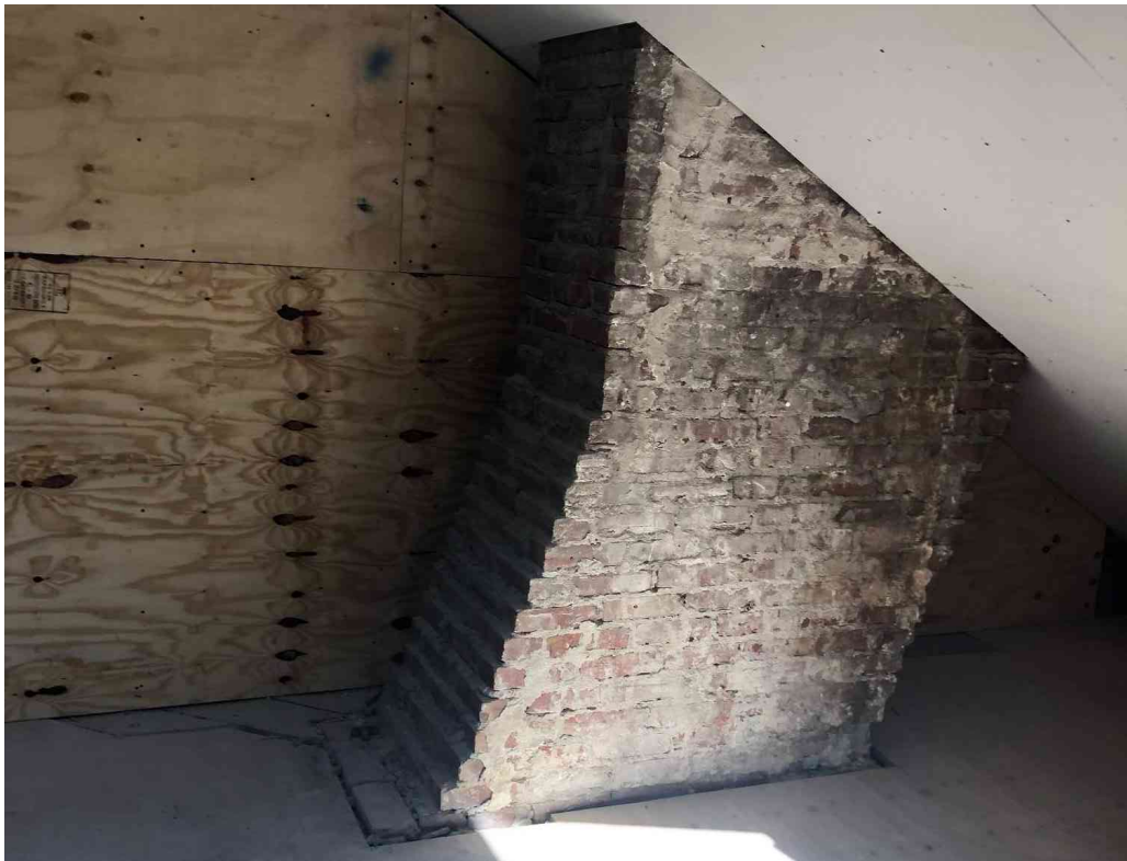
Corbeled chimney in the attic
